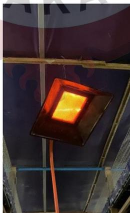
**Gambar 2.14** Heater jenis *gasolec*.
