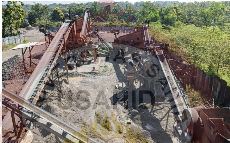
Gambar 2.11 Stone Crusher PT. Prima Stone Persada
